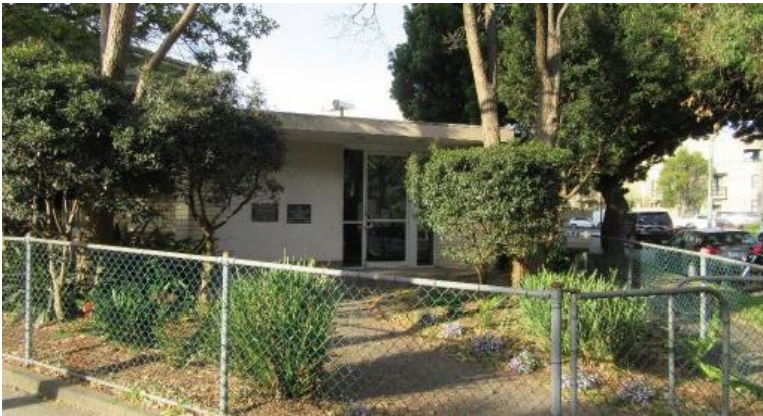
Figure 7. 17A Dadley Street, Alexandria. Photo: TKD Architects
